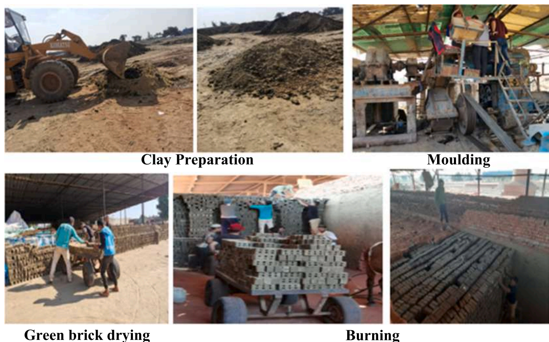
Fig. 1. Brick Manufacturing Incorporating Leachate.
